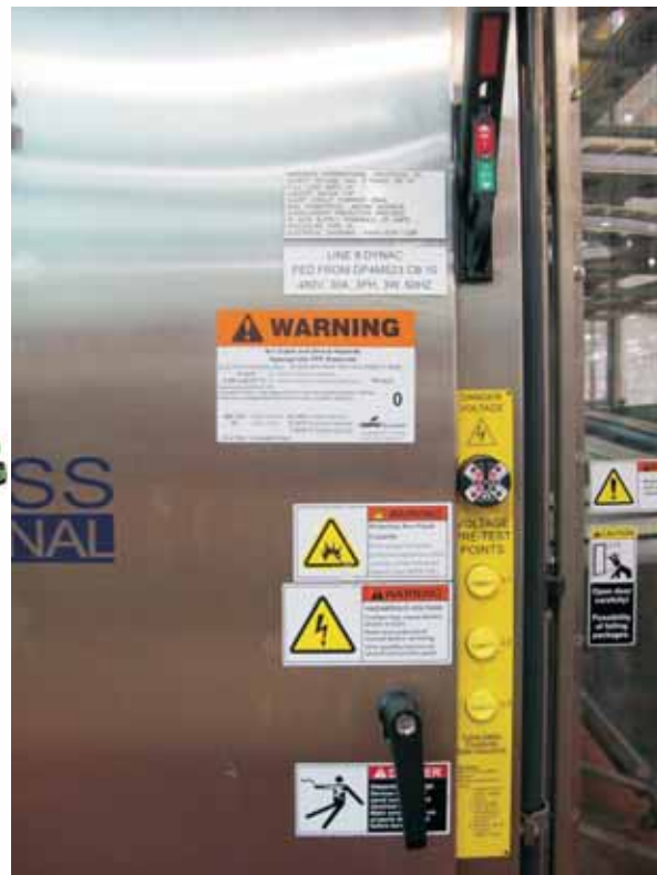
Fig. 6 Installation of a voltages indicator and voltage portals on a typical 3-phase panel.
