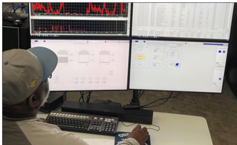
Figure 1. An operator at ExxonMobil's Resin Finishing Plant monitors the plant's operations using the new Open Process Automation console.
