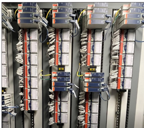
Figure 2. ExxonMobil's new Open Process Automation control panel in Baton Rouge: streamlined and scalable, with standards-based, open technology enabling innovation at a faster pace than existing systems.
