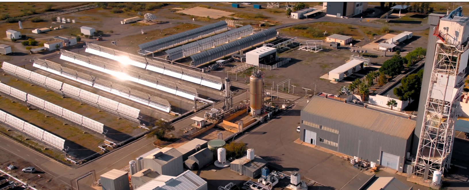
Figure 1. The Plataforma Solar de Almeria TCP-100 facility showing the parabolic trough collectors (PTC). Mirrors focus solar energy on a collection line through which thermal fluid (oil) runs and is heated to about 400 degrees C (752 degrees F), which makes steam to run turbo generators.
