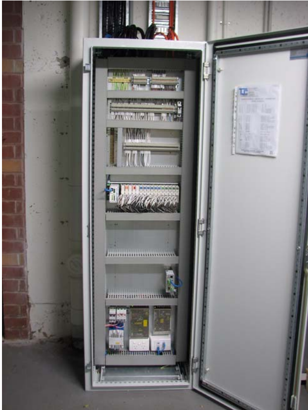
PID-maintained positive air pressure keeps airborne germs out of the operating room.
