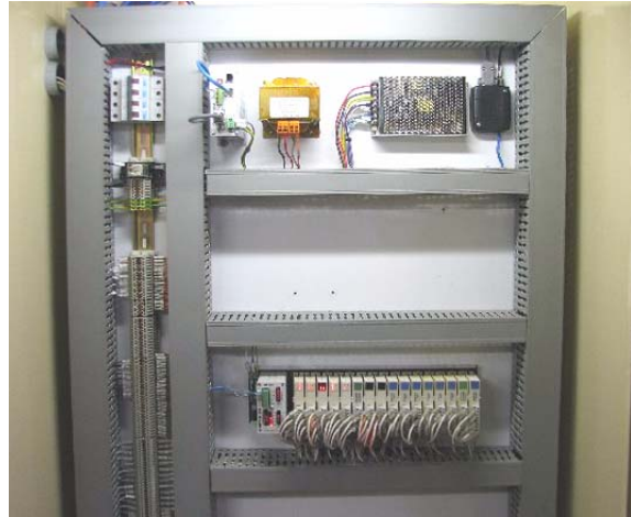
MAs are replaced with SNAP PACs without having to touch any remote I/O or sensors.
