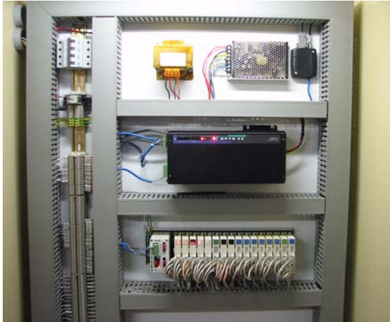
MAs are replaced with SNAP PACs without having to touch any remote I/O or sensors.
