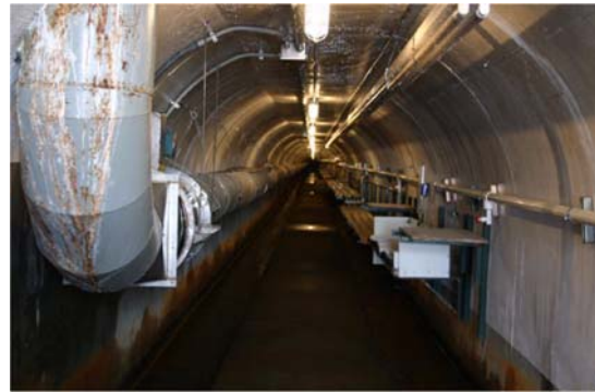
Interior of one section of the LMDT
