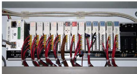
*AIS designed a process control and data acquisition system that includes analog, digital, and high density I/O that controls the thickness profile for the polypropylene sheets.*
