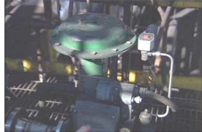
Depending on the industry and the time specific implementation, these assets alone can be somewhat overwhelming. A typical mid-sized oil refinery, for example, may have over 2,000 control loops, each with a sensor, controller, and valve.
