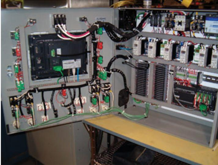
Once the test station was built and delivered, requests for additional analog input requirements were easily met with the extra expansion slots available on the DL06 PLC. Another post-delivery enhancement was the addition of e-mail alerts, sent from the **C-more** panel to notify personnel of failures and other events. A duplicate system was built to meet the increasing demand for customer-specified life cycle testing.
