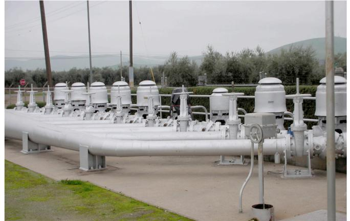
**Irrigation pumps deliver water to customers in the higher elevations to the east of the canal.**
