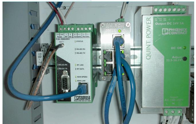
A Phoenix Contact radio and power supply mounted in a control cabinet.
