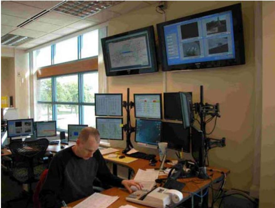
**Figure 1:** Video from 32 remote sites is sent via wireless to the central control room at the Madison Water Utility in Madison, Wisconsin. The video uses the same wireless link as the SCADA and access control system, and the video images appear on a Wonderware HMI system.
