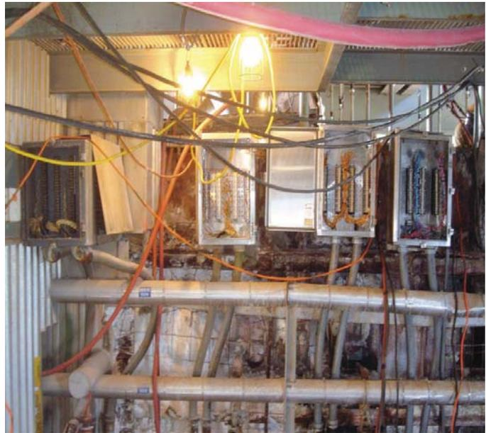
*Figure 2. Hundreds of thermocouple wires are routed to these junction boxes, mounted outside the boiler.*
