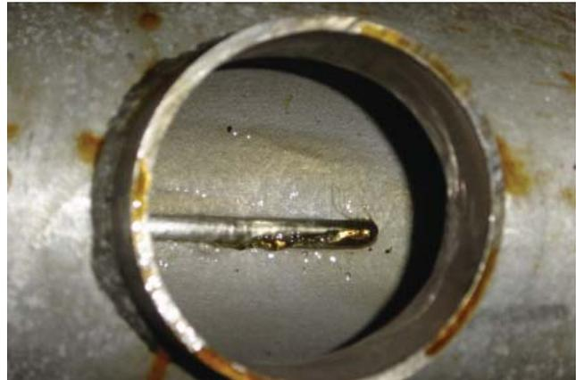
*Figure 3: Looking down through the access hole in the pipe, this photo shows the end of the custom thermowell, lying horizontal. During normal operations, the end of the thermowell is submerged in 1-1/2 in. of molasses.*
