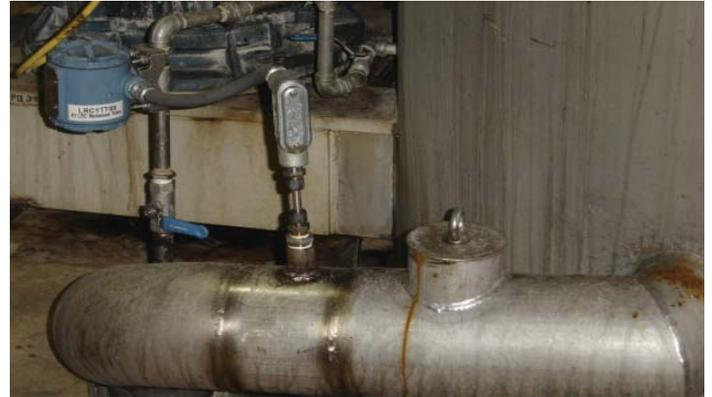
*Figure 1. This six-inch pipe carries molasses from a centrifuge to a storage vessel. A custom thermowell (at the center) was made from 3/8-in. stainless tubing to house a WORM flexible RTD sensor.*
