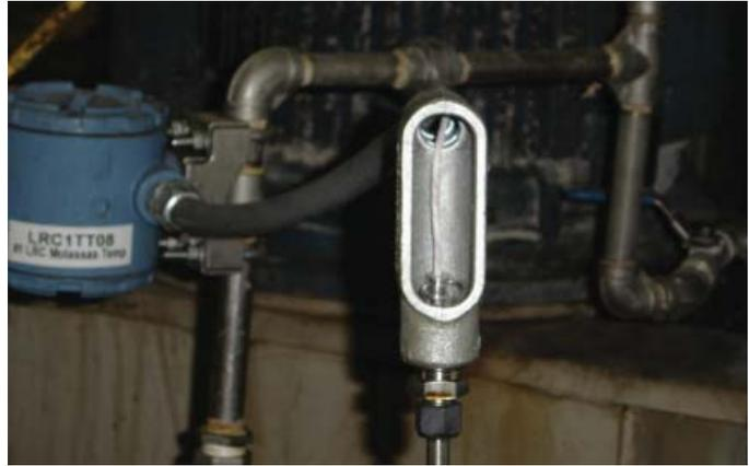
*Figure 2. The stainless steel tubing connects to conduit. The retainer clip for the WORM sensor is visible at the bottom of the conduit.*
