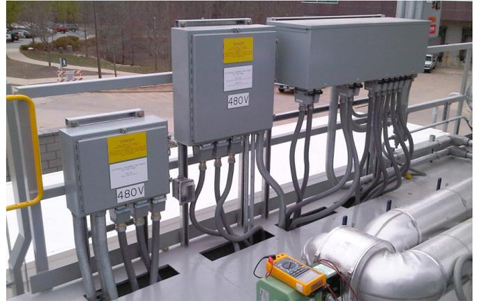
**Power and signal connectors mate to junction boxes mounted on Turbine Inlet Chilling modules, cutting on-site installation time and costs.**
