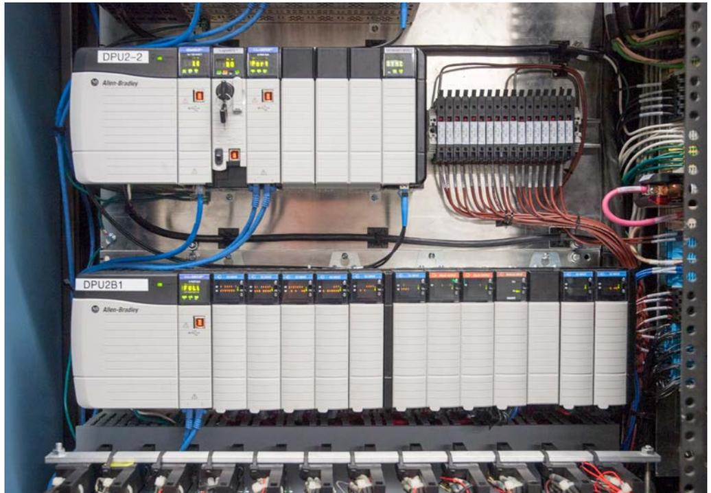
**Figure 3. Time management.** *Upfront planning can reveal many ways to minimize downtime when migrating from an old DCS to a new automation system. This new system allowed existing field terminations to remain intact.*
