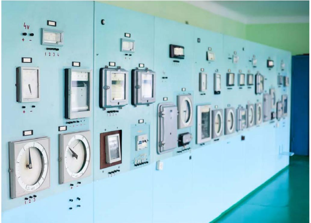
**Figure 4. Old school.** When operator interface panel boards are replaced with modern PC-based HMIs, extensive training is needed to bring plant personnel up to speed.
