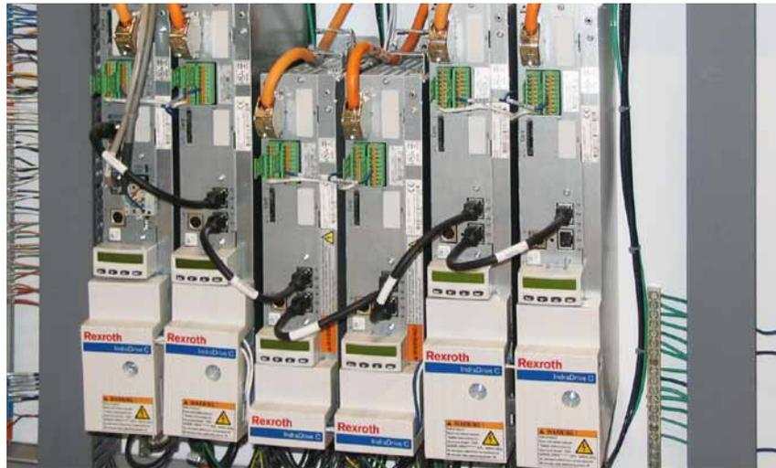
Drive-to-drive cross communications is enabled with SERCOS III: allowing drives to communicate with one another without adding time delays and control processor overhead by going through the master.
