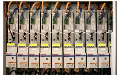
Using dual loop control, Rexroth's IndraDrives provide tight control of the actuator positions, which allow for minute changes in the gap distance.
