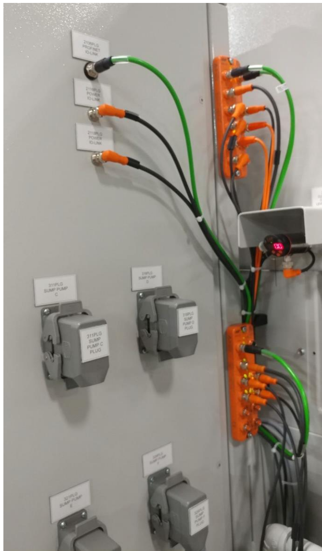
External sensors now plug into IO-Link master modules external to the enclosure. This reduces the number of entries into the enclosure from up to 16 devices to 3 connections for power and PROFINET signal.
